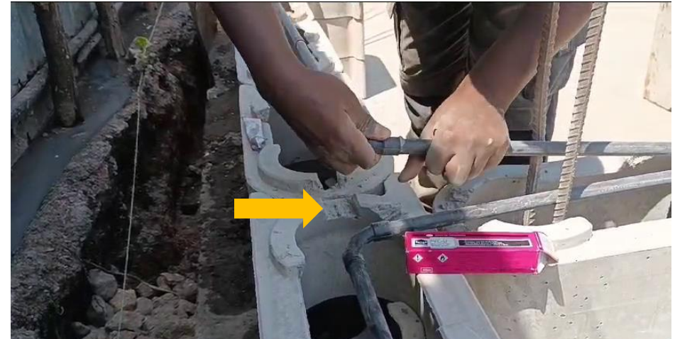
Electrician cutting grooves for conduits to pass through TwistBlock walls.
