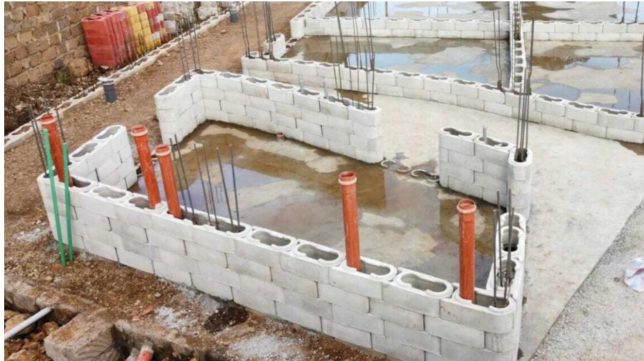
Toilet vent pipes can be slotted into the walls.
