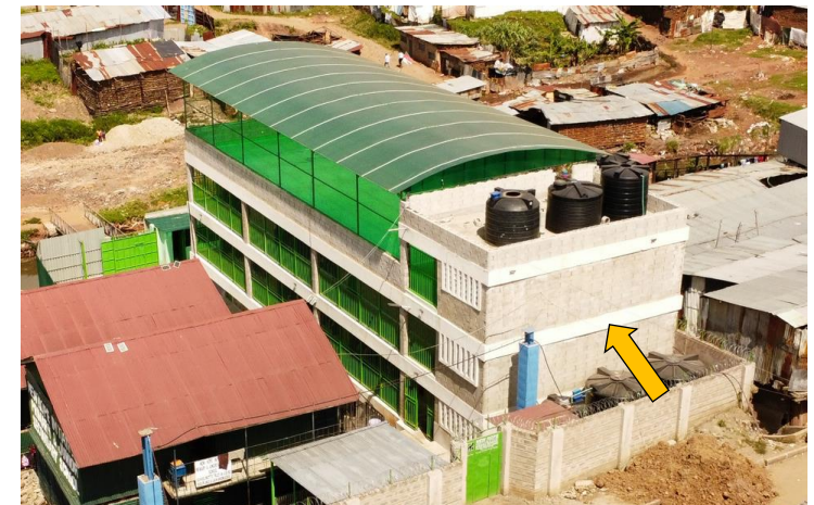
Visible ringbeam and slab edge when using conventional formwork.
