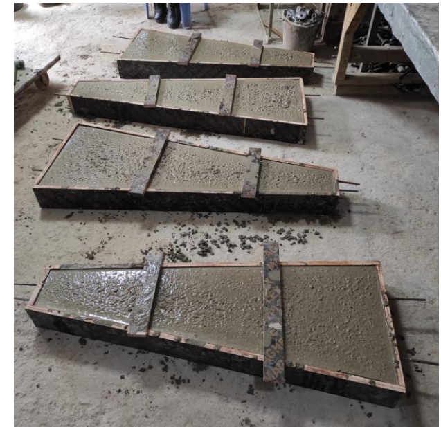
Reusable formwork for pre-cast stairs showing rebar and tread inserts.
