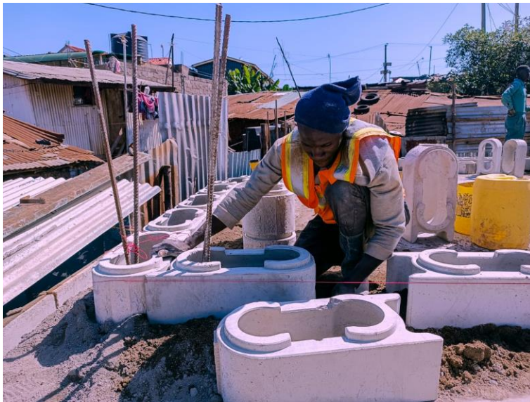
Filling the first layer of TwistBlocks with cement helps the foot of the wall bind with the slab.
