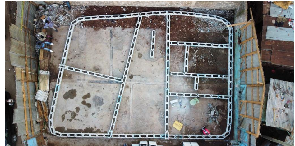
Step C5: test layout of the first course of TwistBlocks to verify the layout fits correctly.
