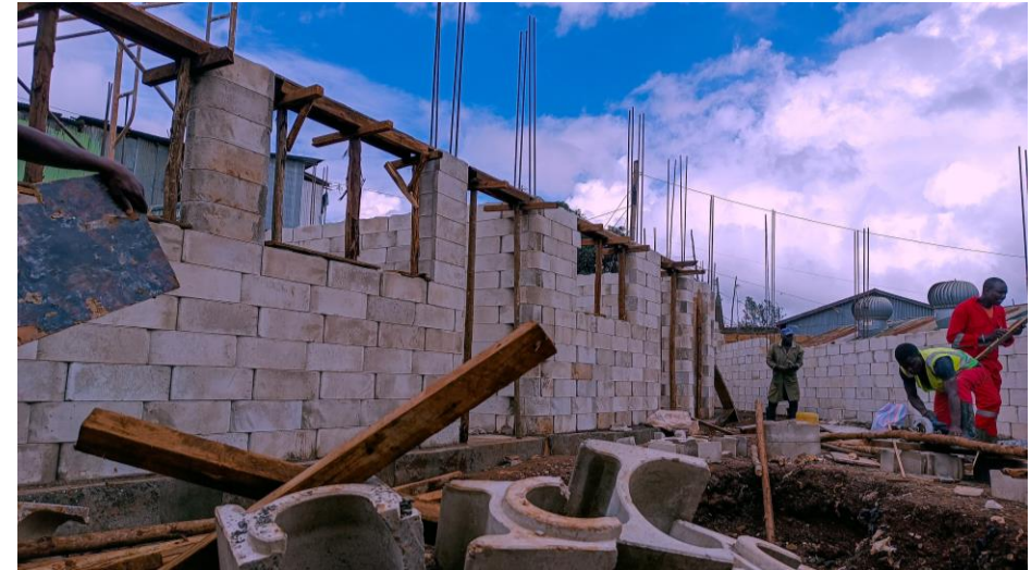
Props supporting the lintels.
