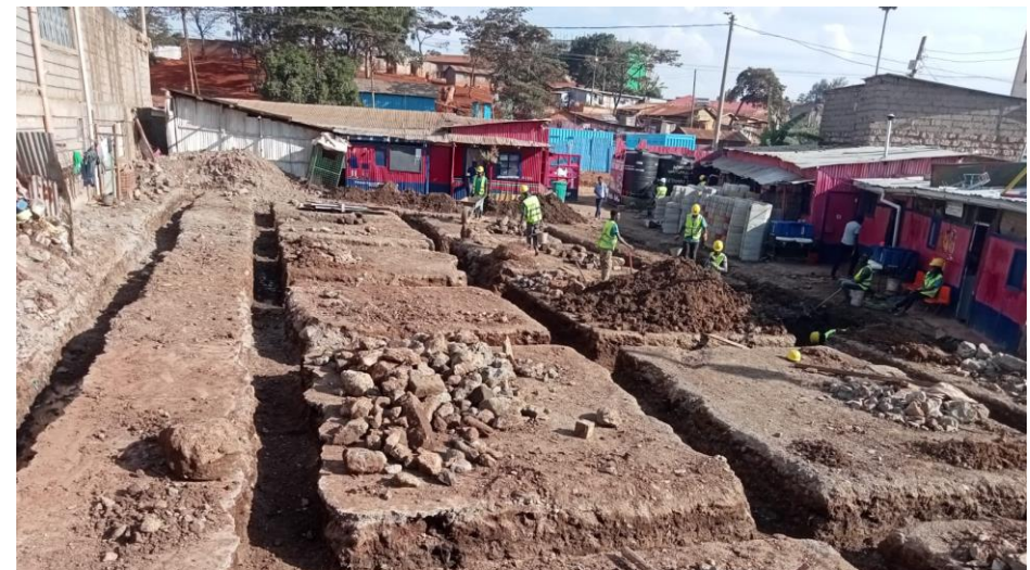
Step D1: Digging the foundation trenches according to the TwistBlock layout.
