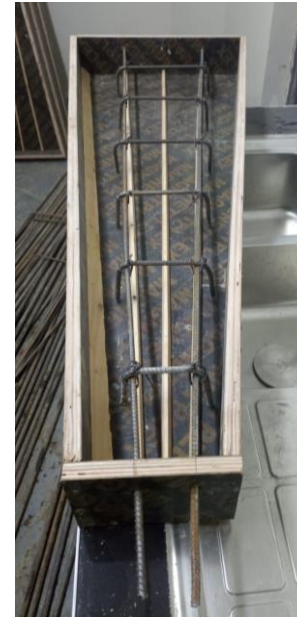
Reusable formwork for pre-cast stairs showing rebar and tread inserts.
