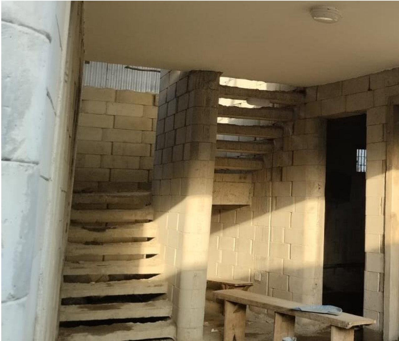
In-situ stairs of 175 x 250mm with a 75mm gap.
