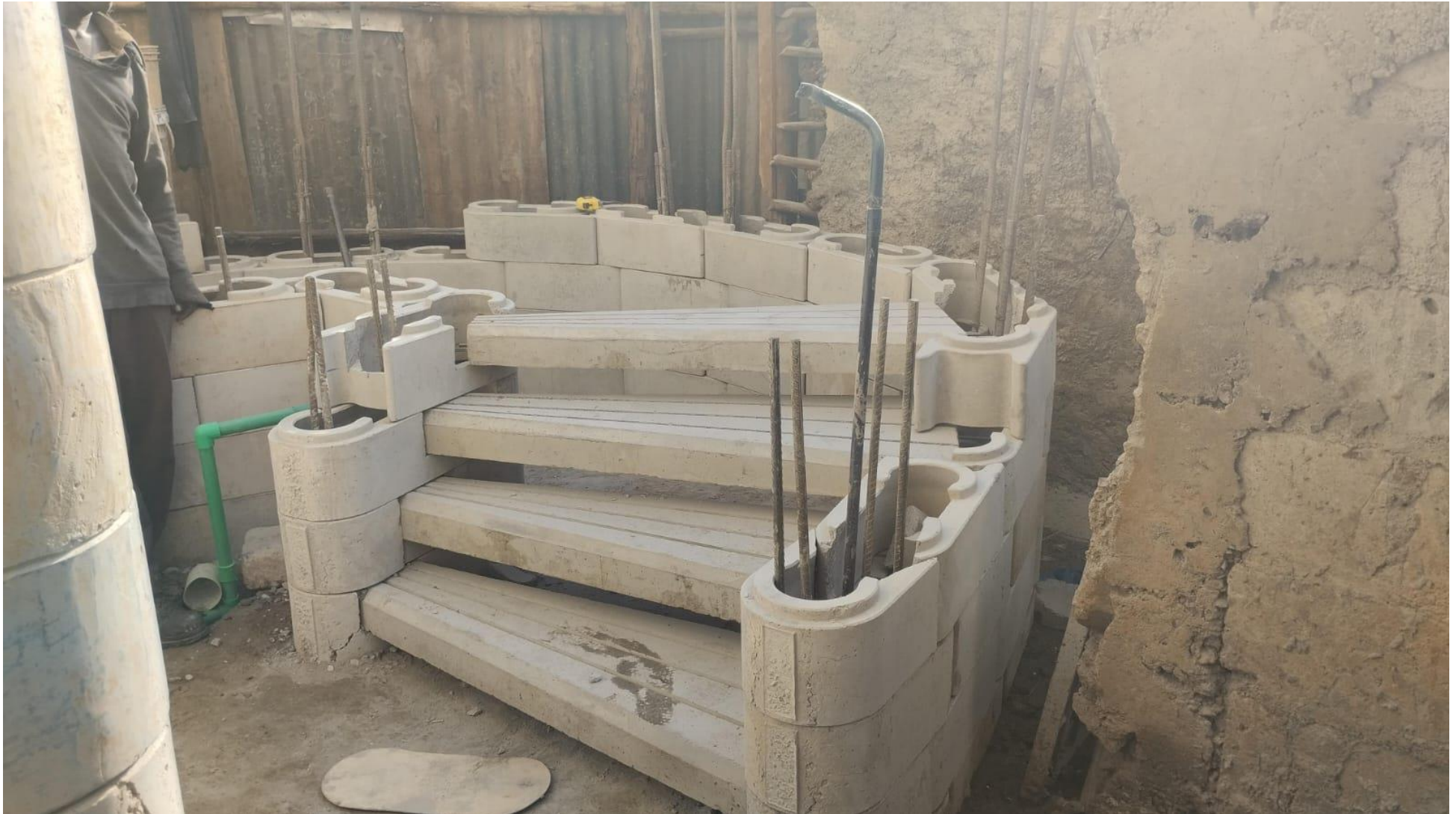
Pre-cast spiral staircase in progress.
