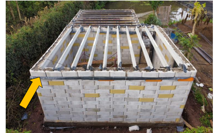
Plastic sheet strip used as “formwork” to support the concrete during casting.
