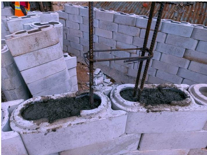
Type two column in progress: concrete should be poured and vibrated every 6 courses. Note – save on concrete and use timber inserts to only fill the ½ of the blocks around the steel.
