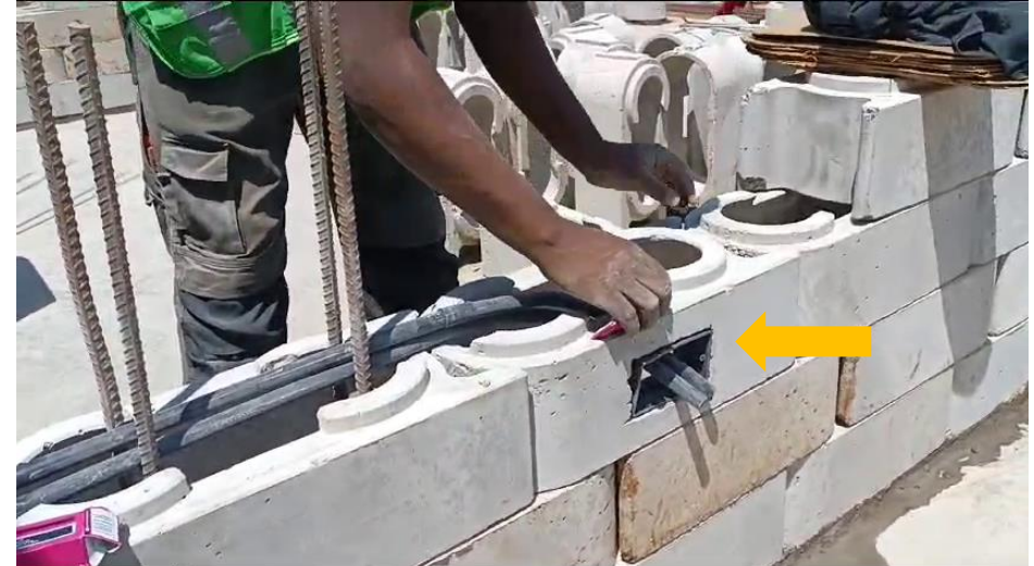
Openings are cut into the face of the TwistBlocks to receive electrical fittings.
