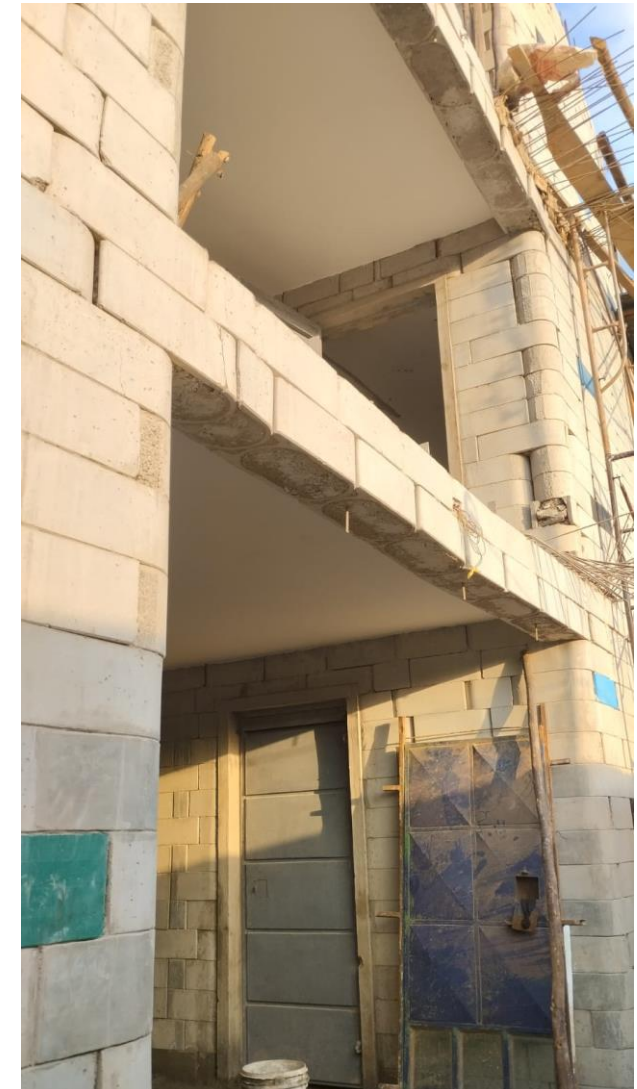
(right) TwistBlocks used at a floating beam position as a formwork for the slab edge.
