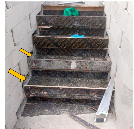
Temporary formwork constructed for in-situ stair casting.
