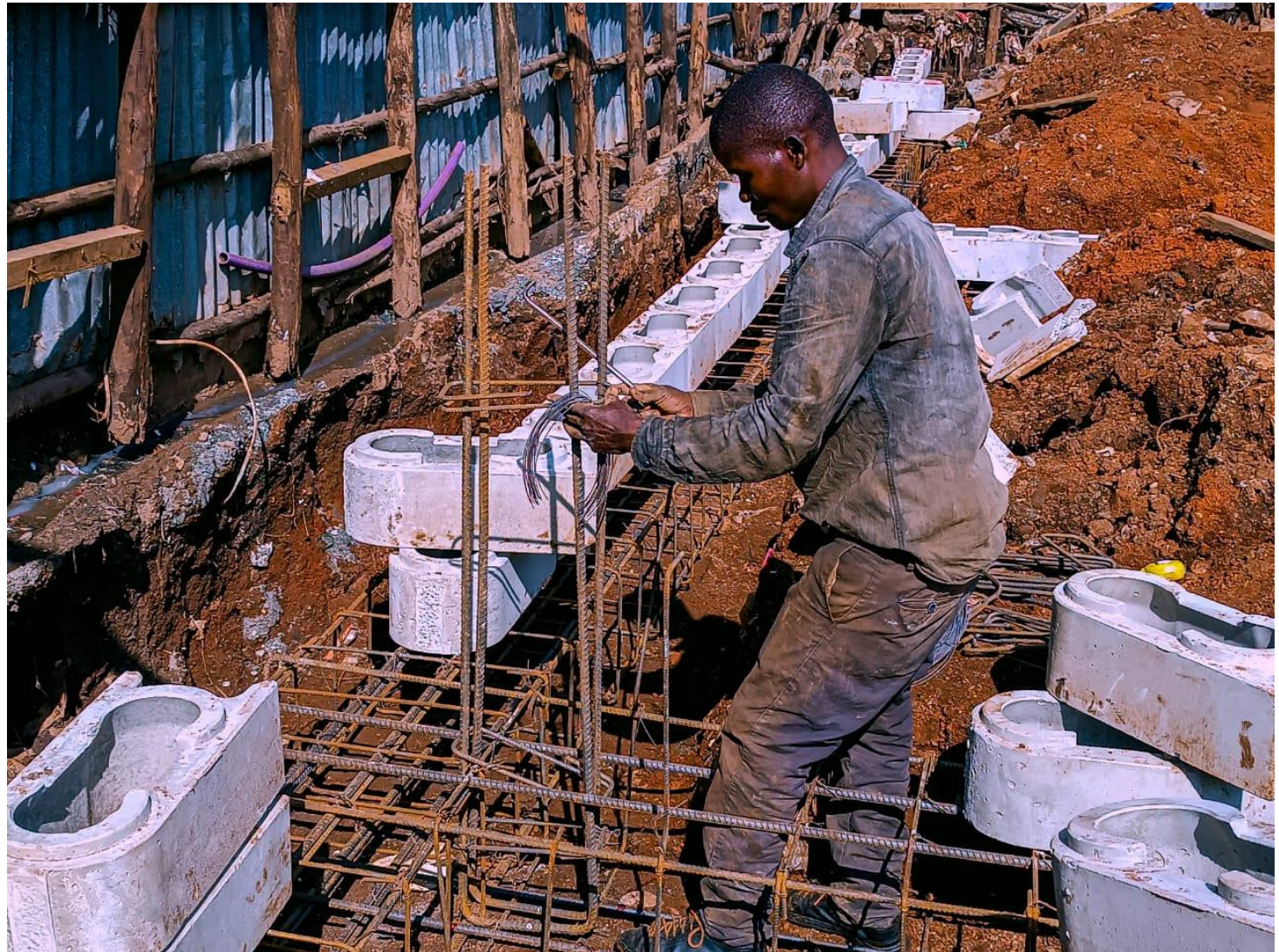
TwistBlock test layout on the foundation steel cages to locate the column positions.
