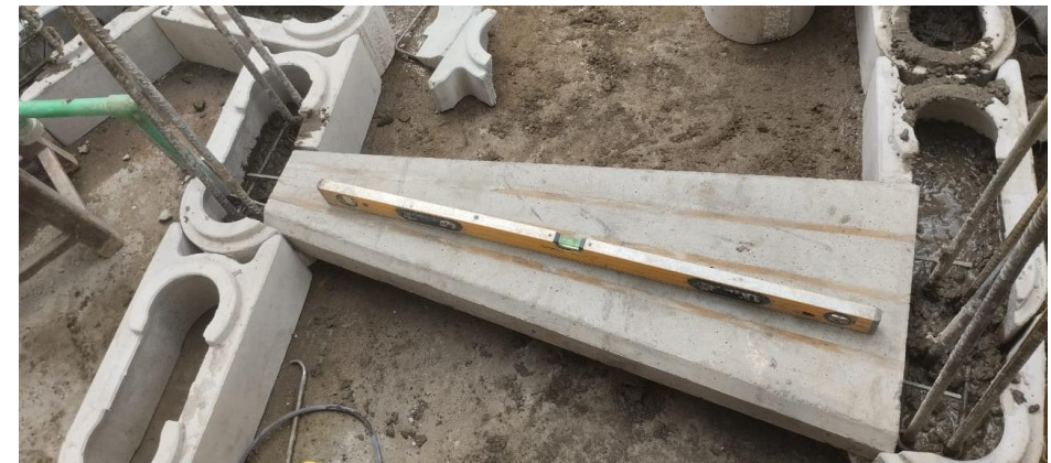
Reusable formwork for pre-cast stairs showing rebar and tread inserts.
