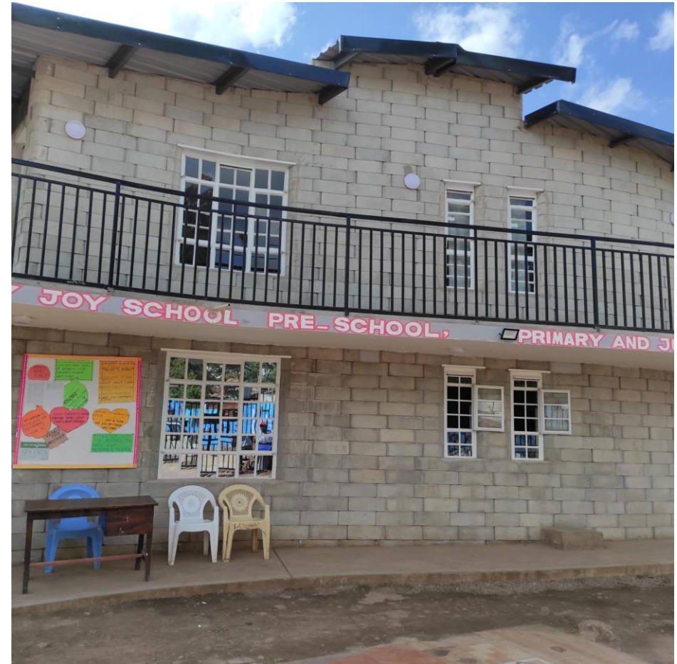
Gabled wall with steel purlins extending through the cut blocks.
