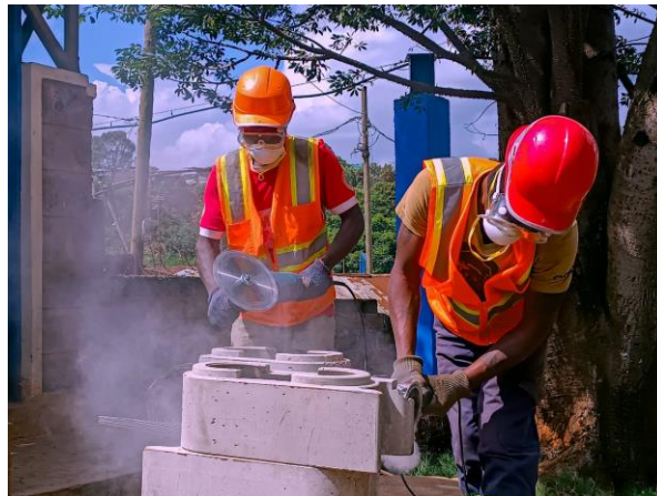
Cutting of blocks using correct protective equipment.
